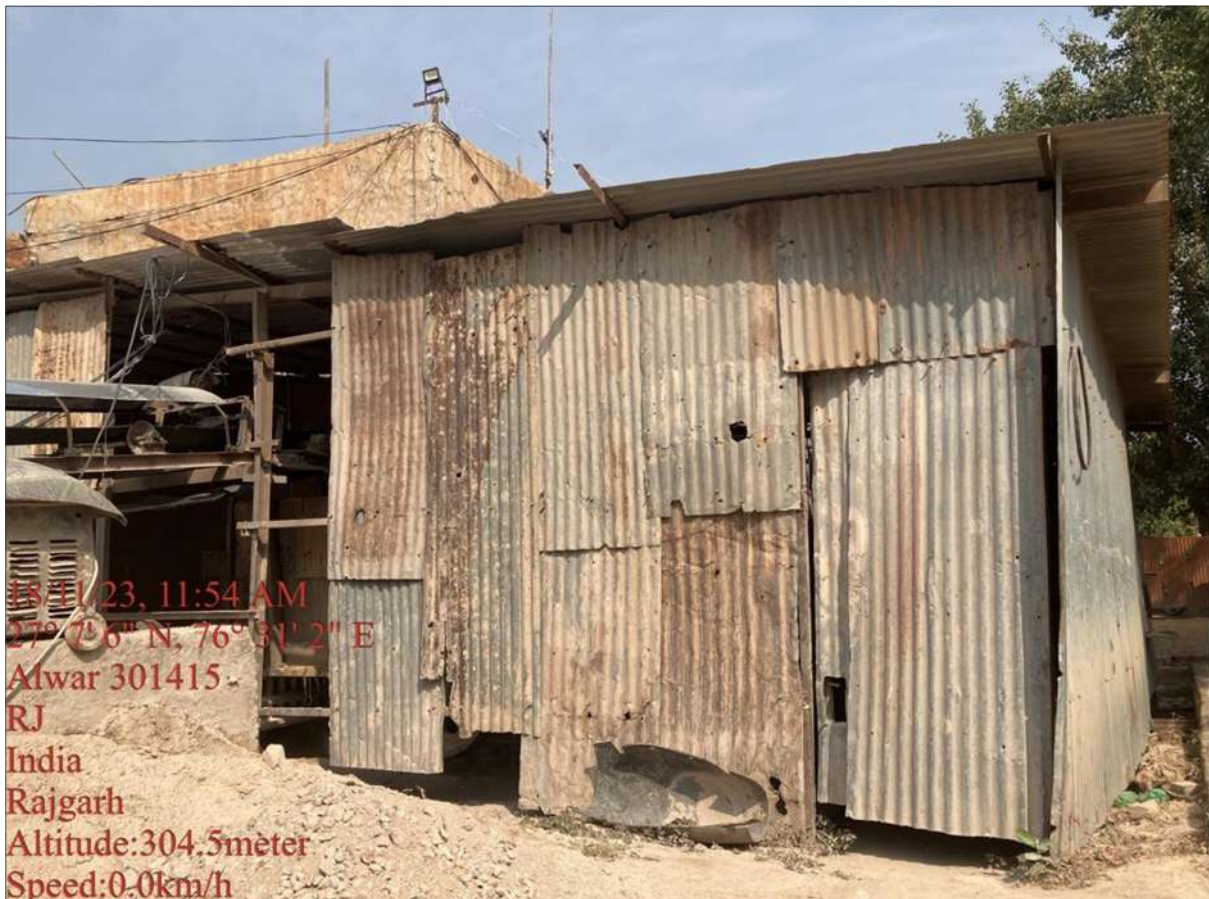
Fig 02: Covered primary crusher (01 No.) and secondary crushers (02 Nos.).
